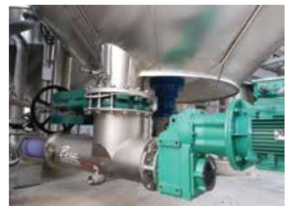
PHC: under-tank flanged pump
